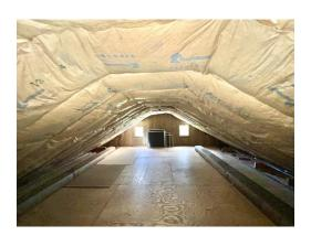
ISSUE The insulation paper backing is exposed.
