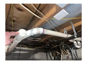
ISSUE The drain pipe is inadequately secured.
