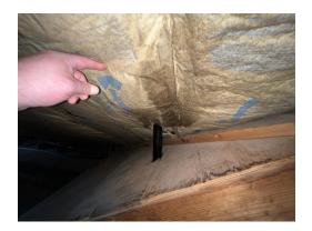
ISSUE There are water stains on the insulation; the insulation is wet. Condensation around the cast iron vent, high
