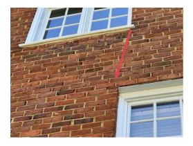
ISSUE There are minor masonry cracks a the lintels.
