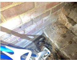
ISSUE There is evidence of active water intrusion at the right side of the basement below the exterior entry door.
