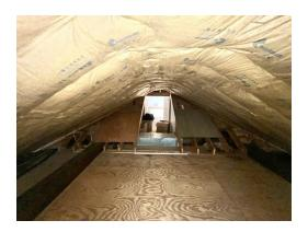
ISSUE There is no attic ventilation system. Evidence of moisture noted on the access door, around the plumbing vent,
