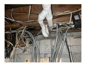
ISSUE The drainpipe is dripping at the rear right of the basement, the moisture appears to be condensation due to
