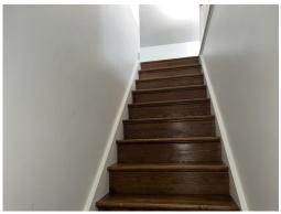
ISSUE The graspable handrailing is not continuous along the basement and loft stairs.
