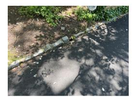
ISSUE The underground drains below the downspouts appear to be blocked, the terracotta drains have a tendency to
