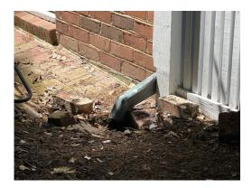
ISSUE The downspout exhaust is not visible; displays signs of blockage.
