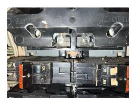
ISSUE Oxidation noted on the terminal bar below the main disconnect
