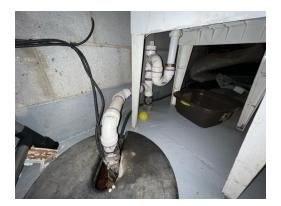
ISSUE The sump pump drains into the municipal sewer system, also the drain line is not adequately sized for the
