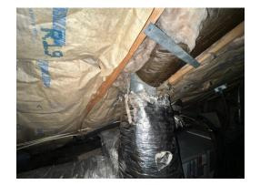
ISSUE The ductwork is separated from the trunk line.
