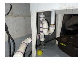
ISSUE The mop sink drain pipe has an "s trap" installed.
